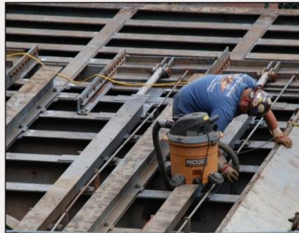
An inside view of a miter gate as it was being inspected and repaired. Wooden panels on the gates have been removed prior to inspection.
