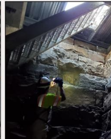
Repairs underway on a gudgeon anchor assembly.
